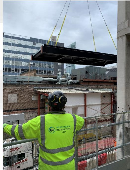
Delivery and installing 8 no pedestrian link bridges in central Manchester.
