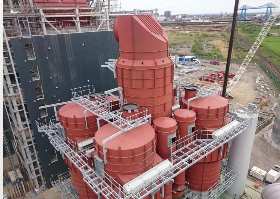
*Installation of 270T Flue Gas Treatment Plant . Sept17 to July18 Location: Teesside .
