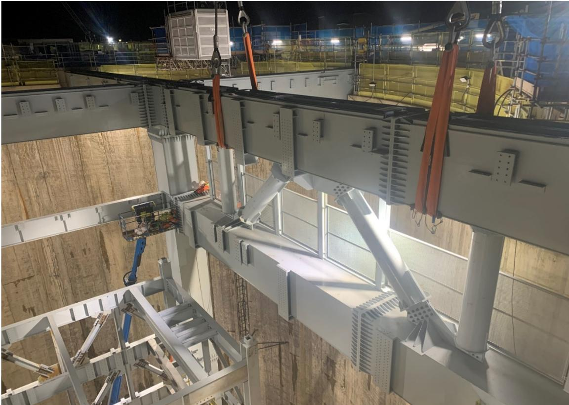
Erection of 1500t of structural steel on a mining project in Yorkshire. TFL have full supply of all labour and plant plus responsibility for H&S and programming.
